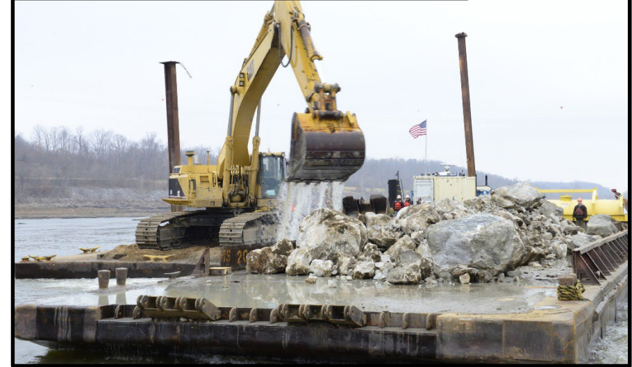
Rock Pinnacle removal at Thebes, IL
